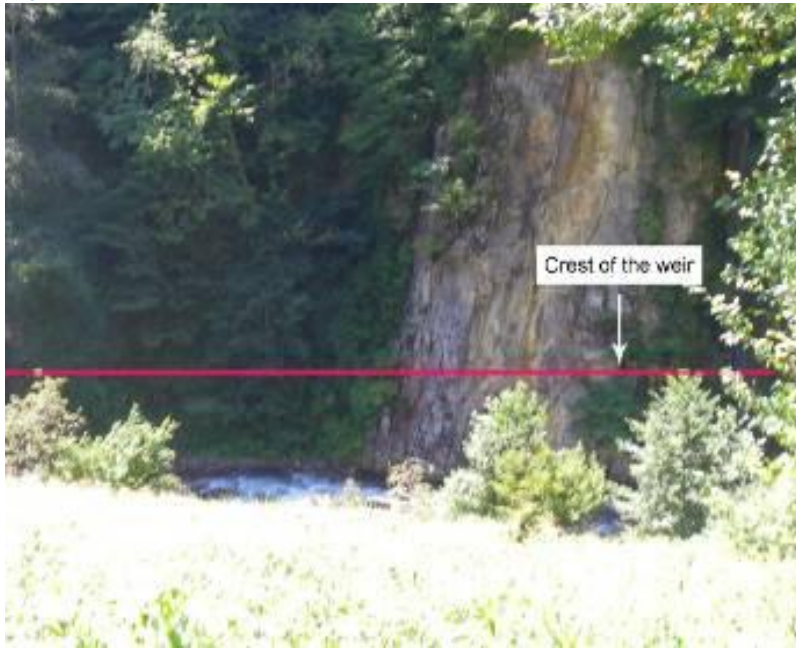
Figure 18.13: Approximate line of crest of Akavreta weir
