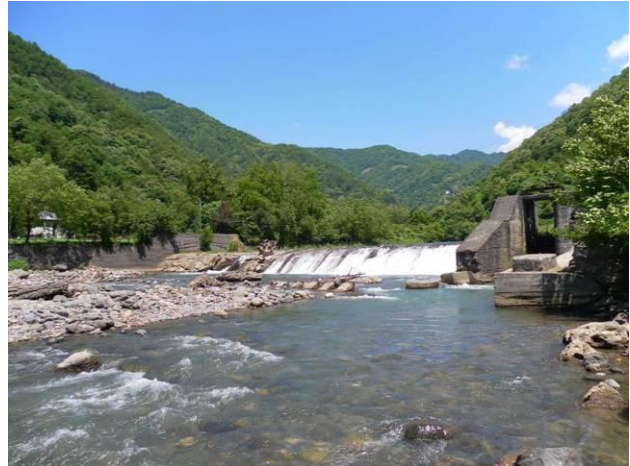
Existing Machakhlistsqali HPP
