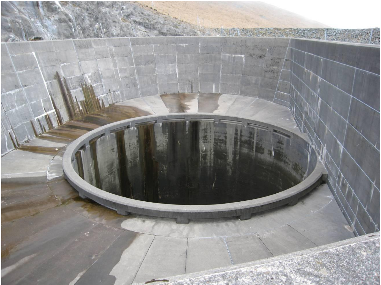
Figure 2.7: Example of surge shaft
