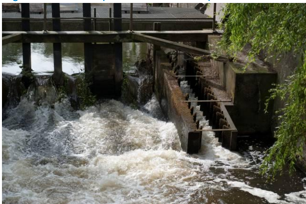
Figure 2.6: Examples of different fish pass structures
