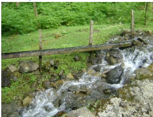
Typical Traditional Irrigation Intake Arrangements: Chvanistsqali Head
