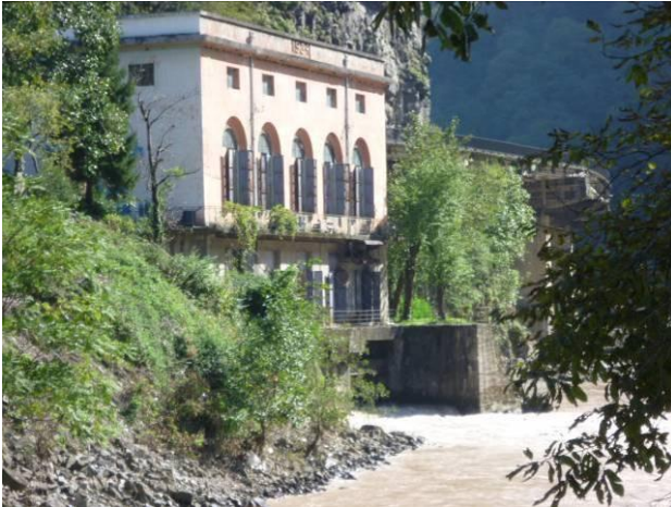
Figure 2.9: Existing Asti HPP Surface Powerhouse
