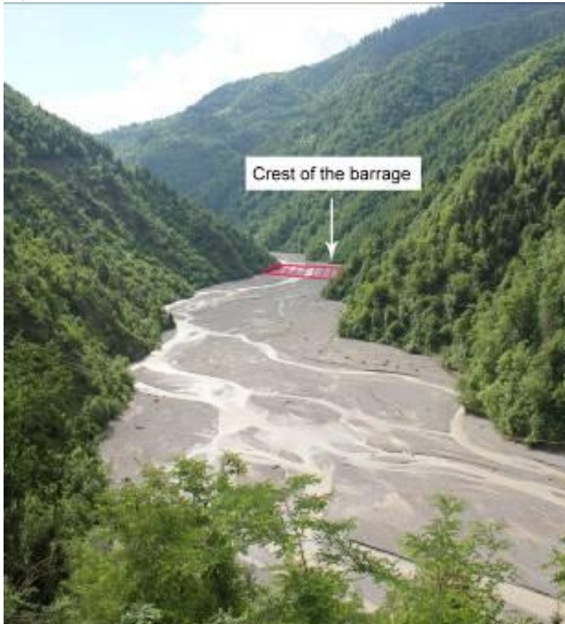
Figure 18.7: Approximate line of crest of Skhalta dam
