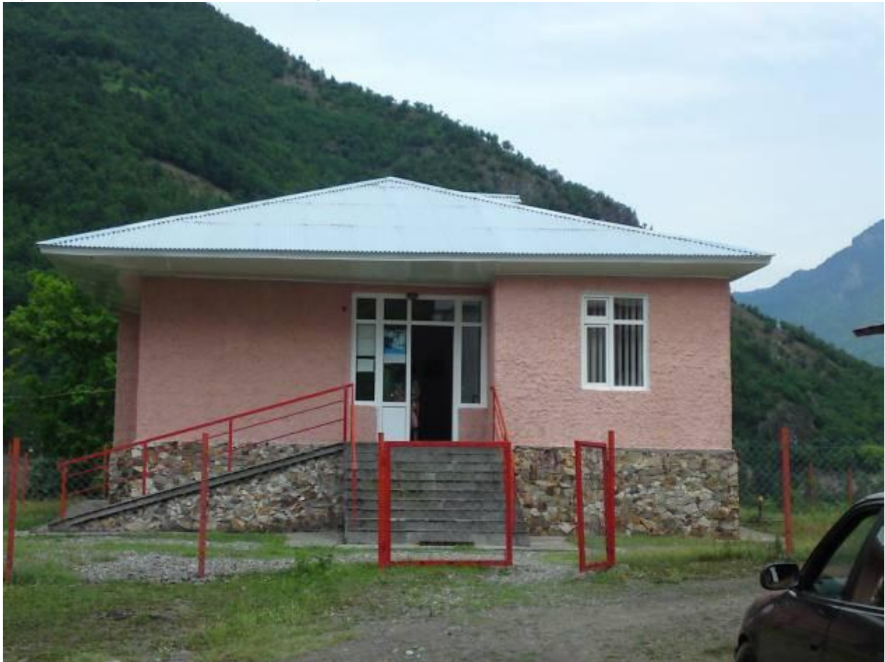
Figure 7.3: Health centre in Zamleti village
