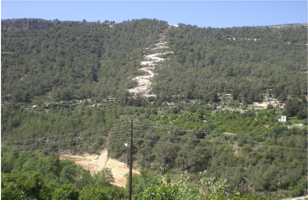
Figure 18.6: Typical view of access road up steep valley side, soon after construction
