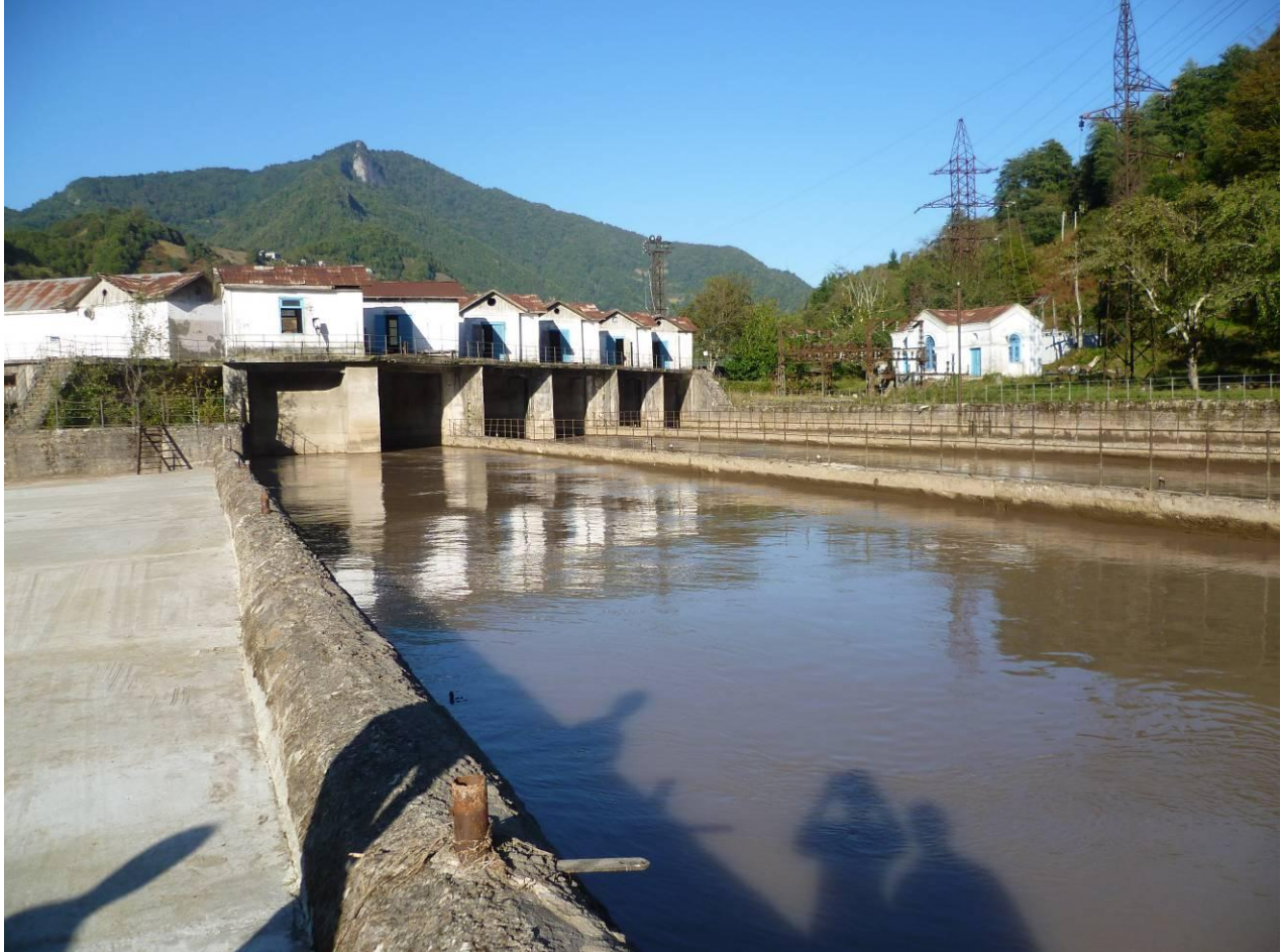
Figure 2.5: Existing Asti HPP Sediment Basin
