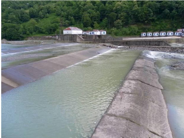
Atsi HPP Weir and Intake Facilities
