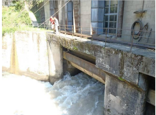
Figure 2.10: Existing Asti HPP Tailrace
