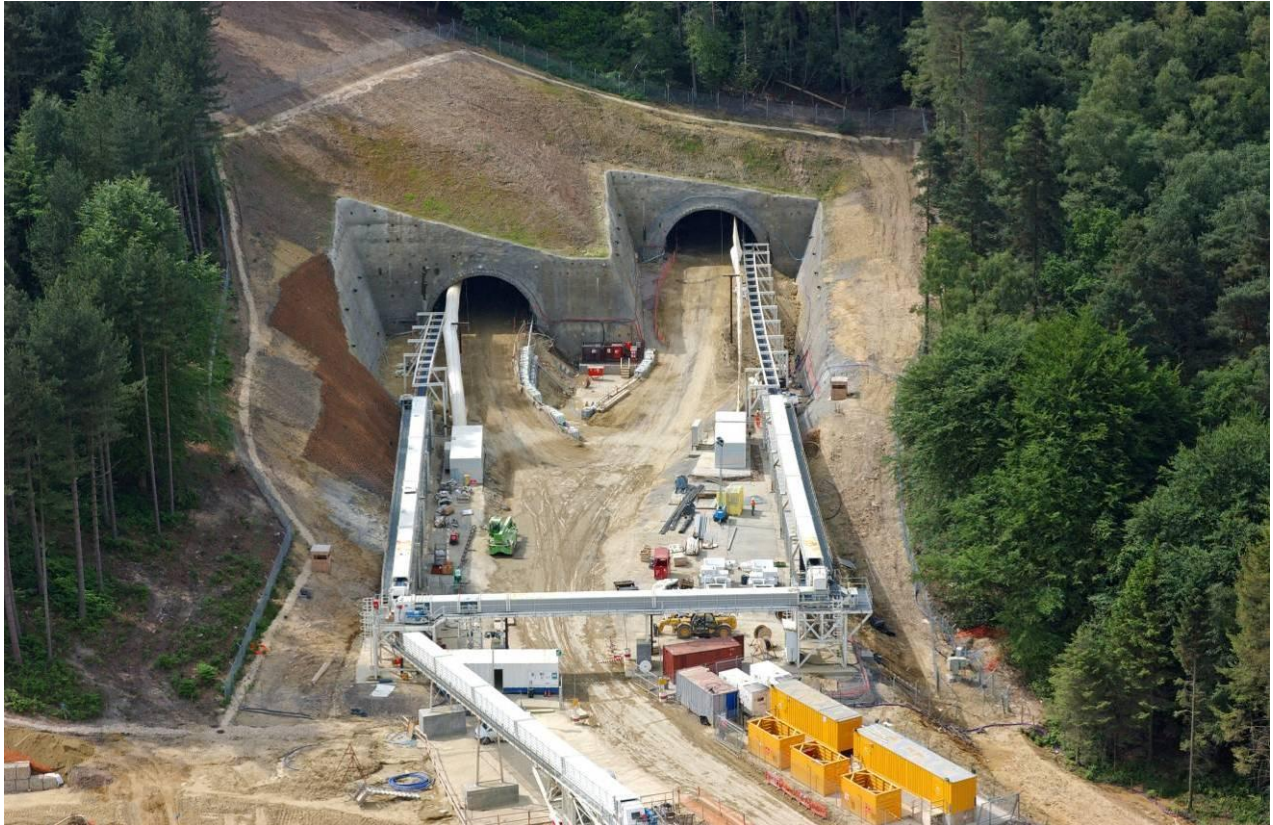
Figure 2.8: Example of Tunnel and Portal Construction
