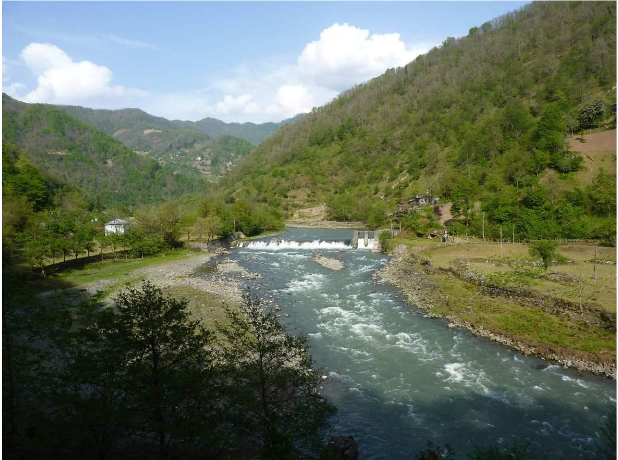
Figure 2.4: Existing Machakhlistsqali HPP Concrete Weir
