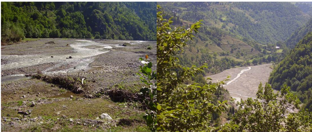
Just downstream of the Skhalta Dam footprint (2013)
