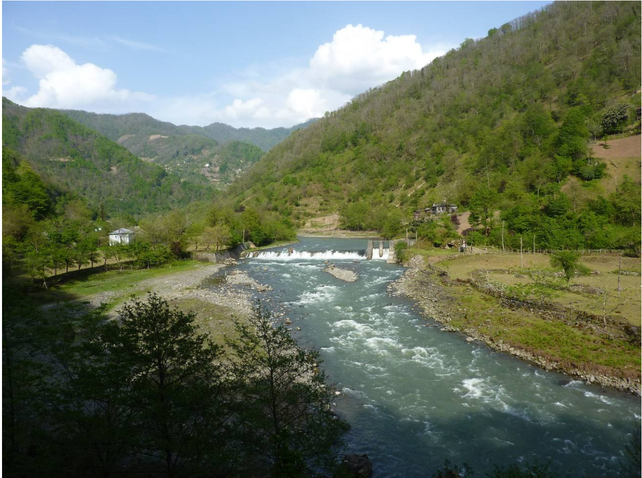
Figure 2.6: Existing Machakhlistsqali HPP Concrete Weir
