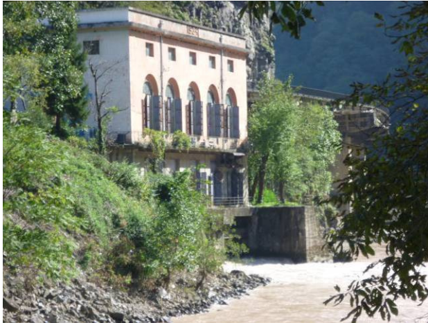
Figure 2.11: Existing Asti HPP Surface Powerhouse
