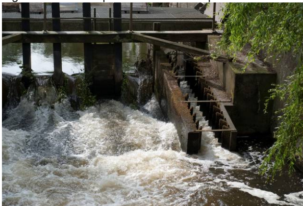
Figure 2.8: Examples of different fish pass structures
