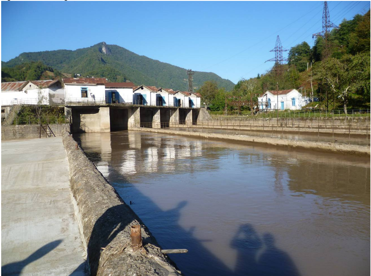
Figure 2.7: Existing Asti HPP Sediment Basin
