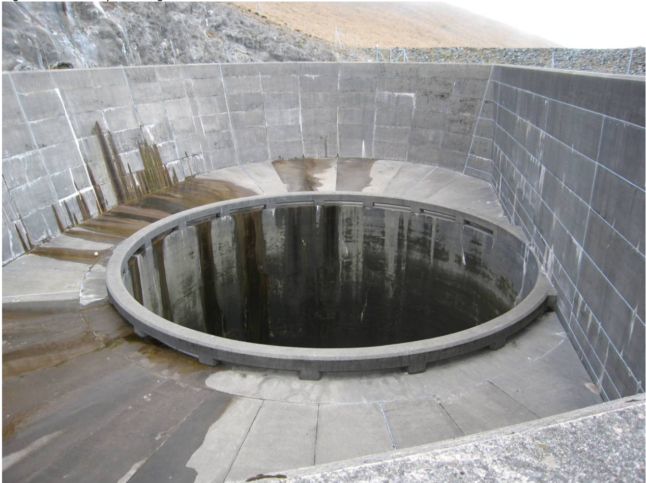
Figure 2.9: Example of surge shaft
