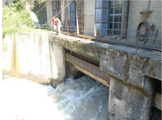
Figure 2.12: Existing Asti HPP Tailrace
