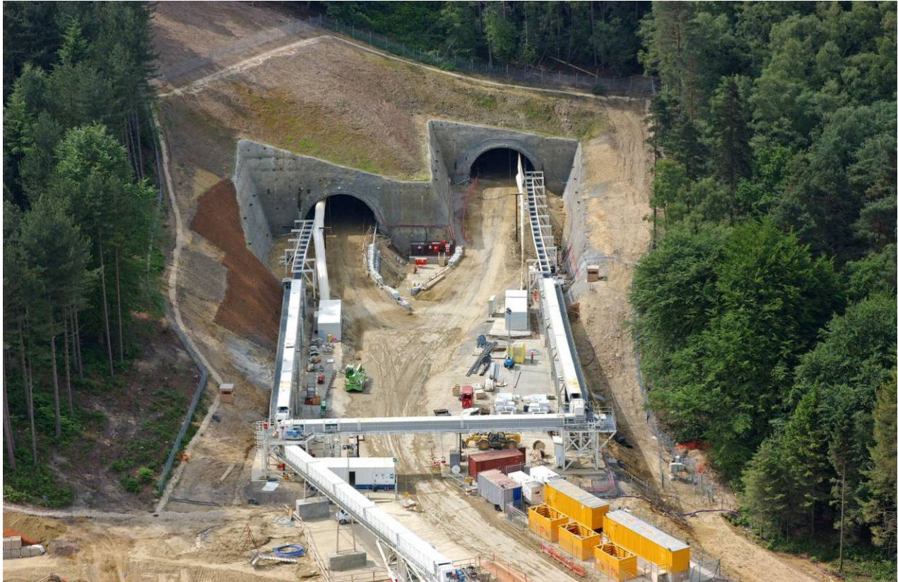
Figure 2.10: Example of Tunnel and Portal Construction
