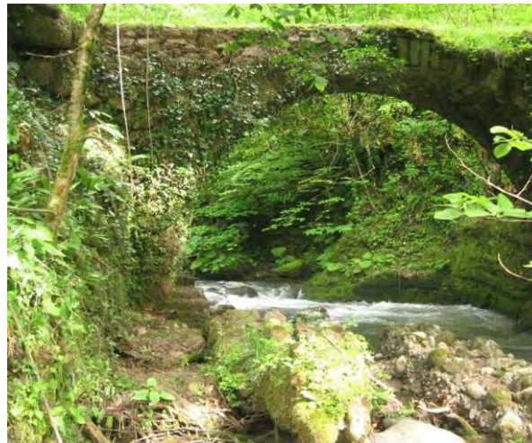
MM66 Historical bridge near Chvani village
