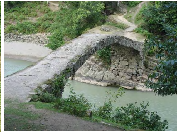
MM35 Bridge in Makhuntseti village
